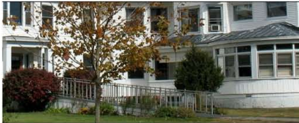
Detail of Existing Ramp
